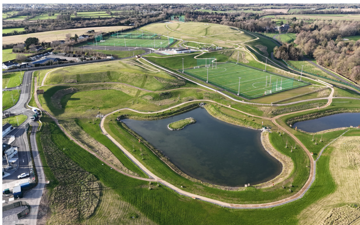
Remediated Kerdiffstown Landfill
