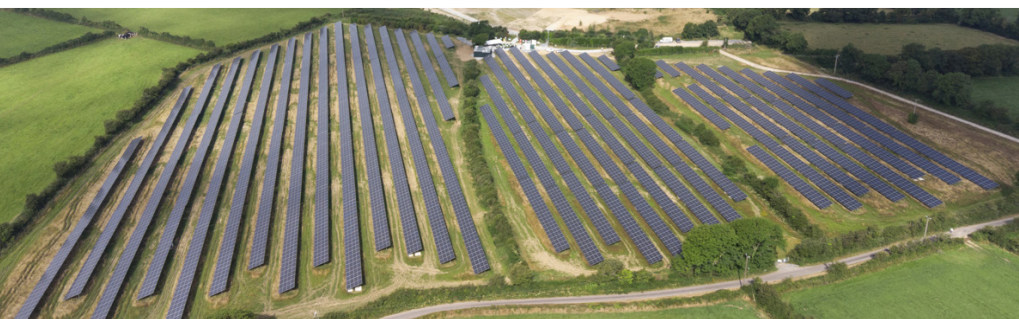
Solar Farm Installation at Licensed Site
