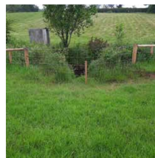
FIGURE 5: Raw water at Glaslough Tyholland PGS after implementing source protection measures.
