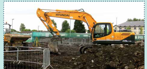
07 Reduce the idling times of plant and machinery through driver training.
