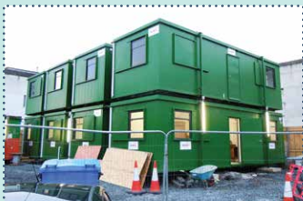
01 Install occupancy sensors in the site accommodation.
