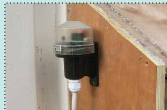
03 Install photocells for security lighting.
