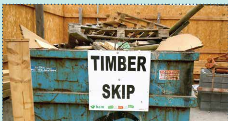
01 Segregate timber and metal on site.
