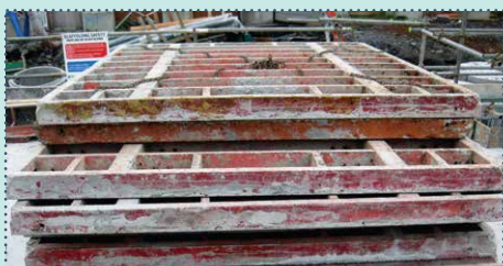
06 Use a reusable shuttering system.
