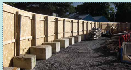
03 Reuse site hoarding elements.
