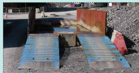
06 Use waterless or recirculating wheel wash systems.
