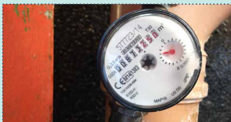
01 Install a water meter to monitor usage on site.
