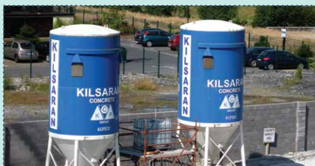
05 The use of mortar silos also reduces water usage.
