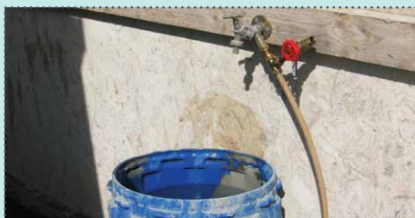
04 Install a tap system and tool washing facility.
